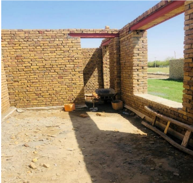
Shelter in the construction phase in Imam Sahib
